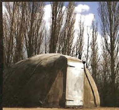
Inventors Peter Brewin and William Crawford visited a refugee camp in Uganda during a tropical storm, and learned firsthand how much safe, semi-permanent shelters are needed. The structures come in packs containing cement-impregnated fabric bonded to the outer surface of an inflatable plastic liner. Photos: Concrete Canvas.
