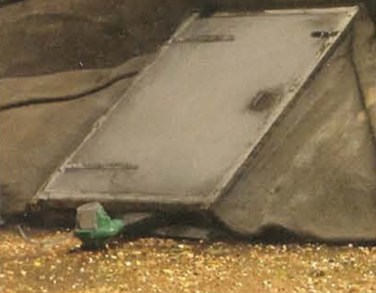
Inventors Peter Brewin and William Crawford visited a refugee camp in Uganda during a tropical storm, and learned firsthand how much safe, semi-permanent shelters are needed. The structures come in packs containing cement-impregnated fabric bonded to the outer surface of an inflatable plastic liner. Photos: Concrete Canvas.
