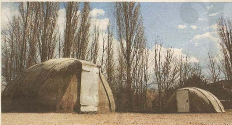
Examples of the 'concrete canvas' tents, invented by Peter Brewin and Will Crawford
