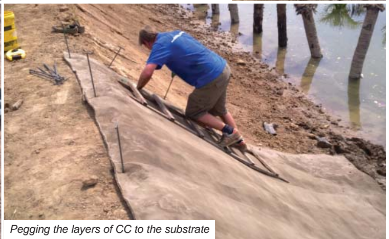
Vertically positioning batched lengths of CC8
