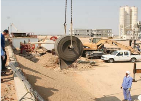
CC4 or CC8 in rolls of 200sqm or 125sqm respectively can be handled & positioned using site plant.
