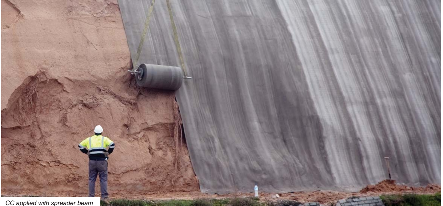
CC applied with spreader beam
