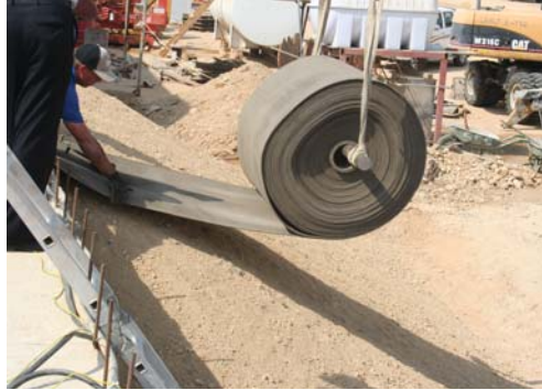
CC is rolled from the slope crest down the slope face, with 100mm overlaps between adjacent CC sheets.
