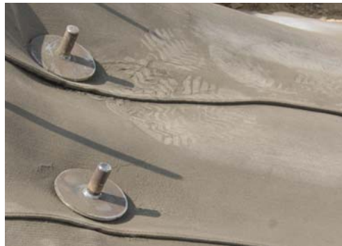
CC is fixed using short nails hammered into the soil. Other fixing methods such as drilled bolts can also be used if rock is present.
