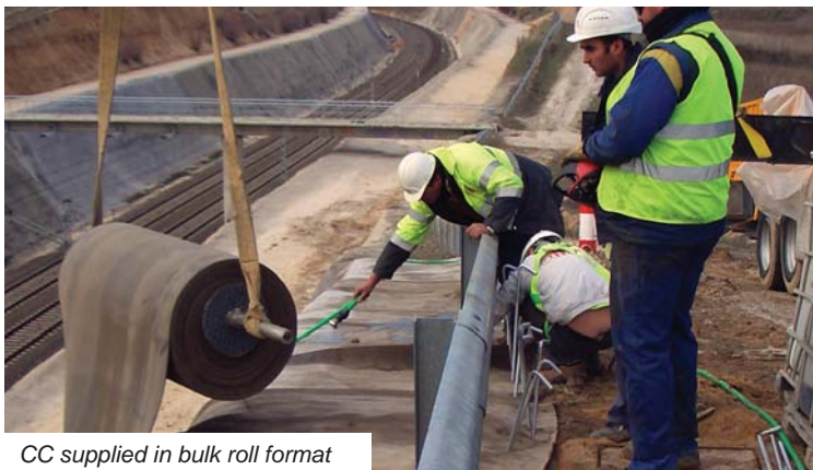
CC applied with spreader beam
