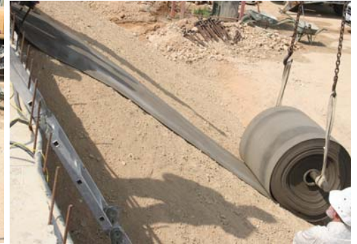
CC is cut to length, depending on the slope size.
