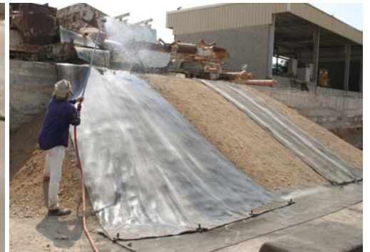
CC is hydrated once fixed into position. Lined drains can be formed from CC at the slope crest and toe.
