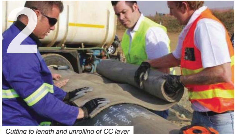
Cutting to length and unrolling of CC layer
