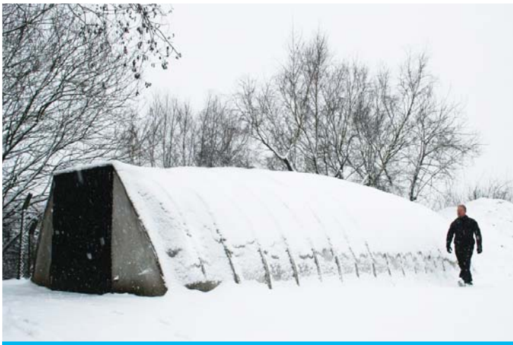
CCS50 deployment, South Wales, 2008
